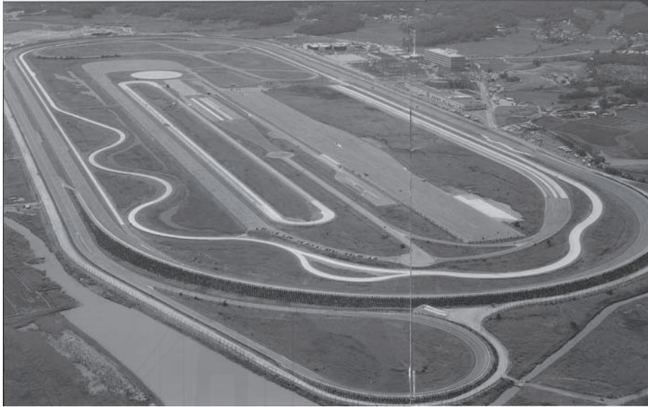
Figure 15.9 View of Hyundai Research Centre at Namyang
